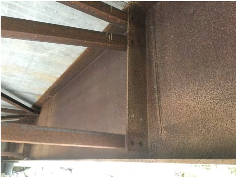
Bolt holes in stiffeners but all bracing welded
