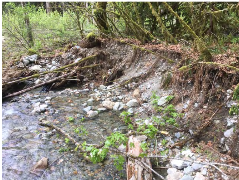
Bank erosion upstream from bridge crossing
