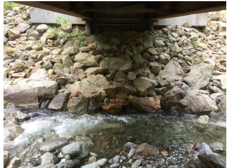
Left Bank Abutment when facing downstream
