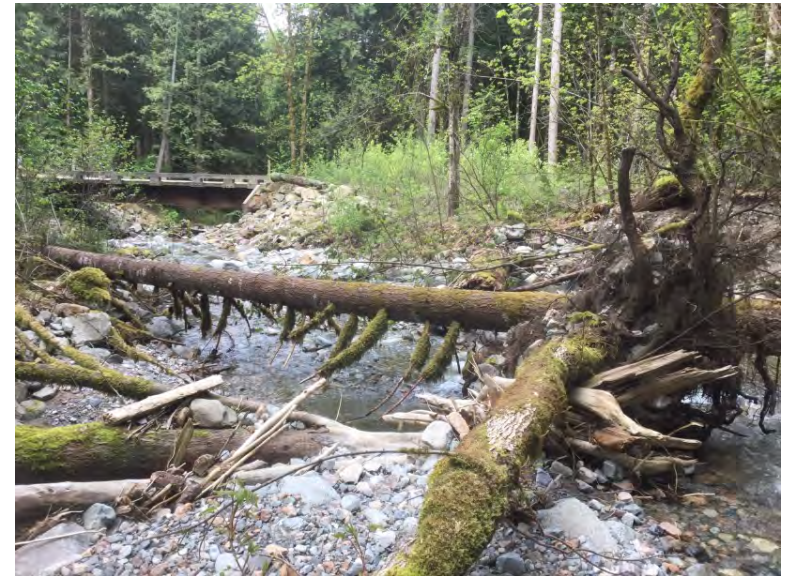
Debris in stream located above bridge crossing
